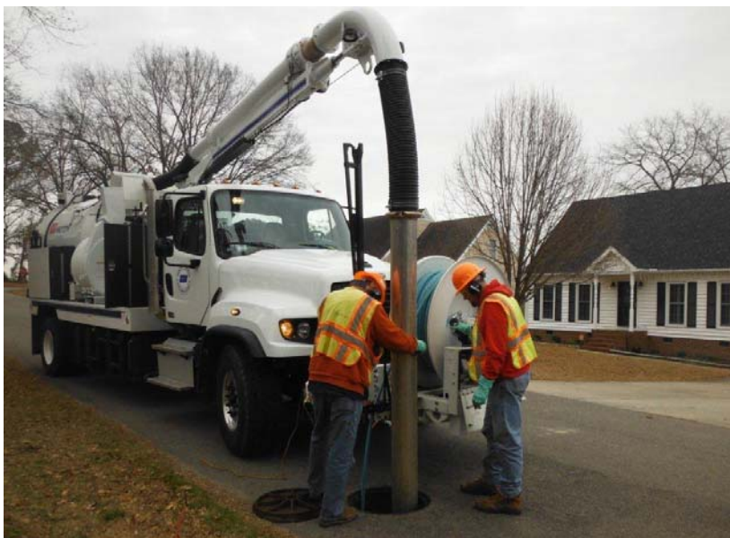
The District uses New Vacuum Truck to Clean Sewer Line
