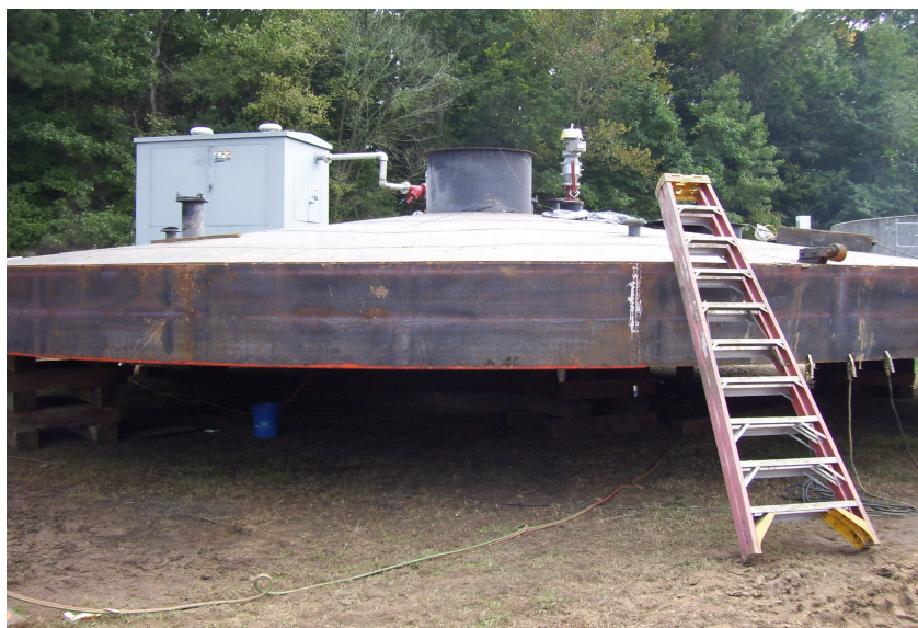
Removed floating Anaerobic Digester cover under repair.
